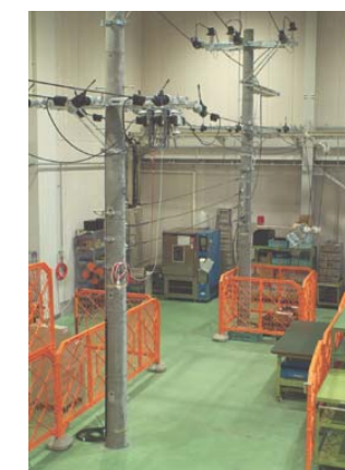
Simulated power pole for electricity distribution line
