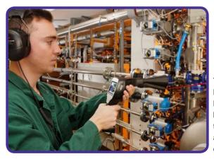
The noise-proof headset enables the leak detection also in EXTREMELY loud ambient. The ambient noise will be faded out, the leakage (inaudible ultrasonic sound) will be transformed to an audible signal. The laser grants an exact locating.
